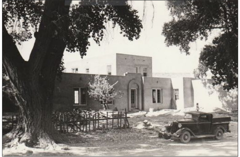
El Refugio under construction, 1942. Photo courtesy of Lynn Mullins.
