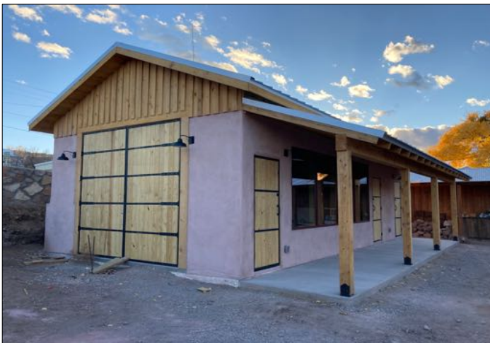
View of the Coach House from the northeast, as of November 28. The large opening is, of course, for the coach itself, fitted with prominent hand-crafted wooden doors and heavy iron hinges. The area in front of the building will be landscaped as an outdoor venue for community events.
