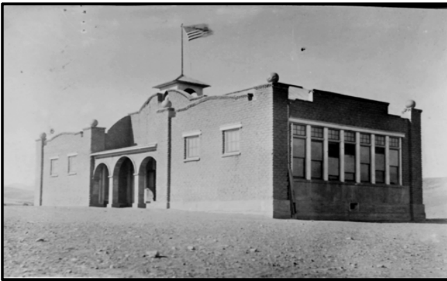
Fig. 7. The second schoolhouse, completed in 1911. Photo Black Range Museum.
