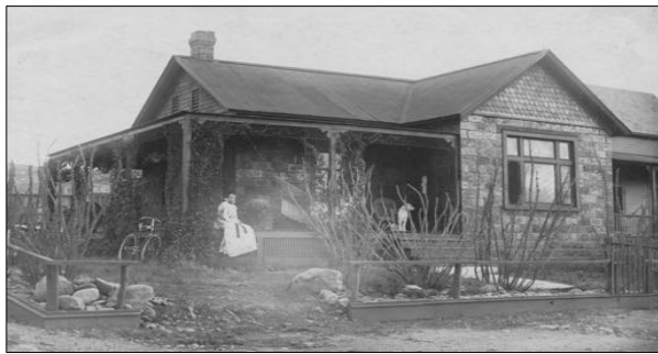
Figure 5. Ninette on porch of the Miller home on Elenora Street, built of black slag blocks.
