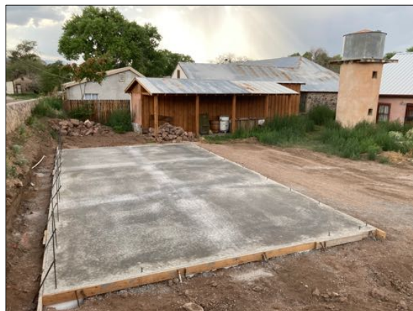
The concrete slab for the new Carriage House, poured August 2.
