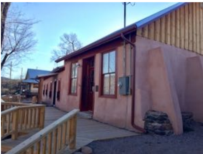
The Black Range Museum, showing newly installed gutters and facia, fresh paint, and handicapped accessibility ramps.
