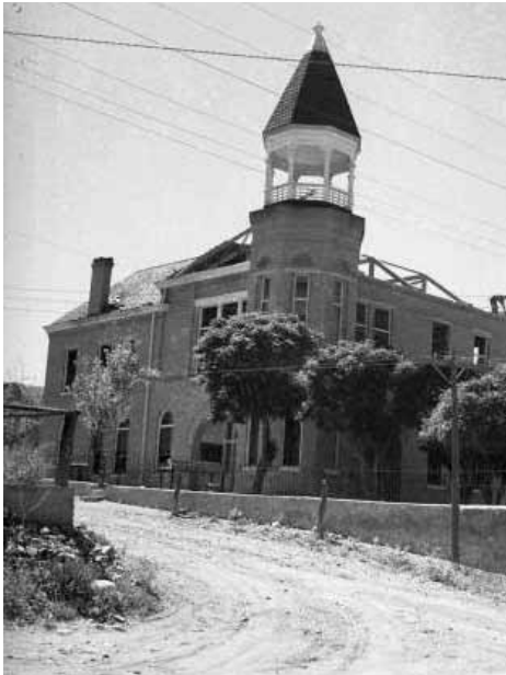
Tear down Begins
