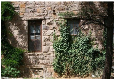
Detail of the Victorio Hotel stonework. Photo www.oldhousedreams.com.
