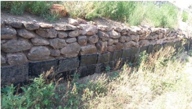
Photo 6: Slag blocks in retaining wall of Disinger house
