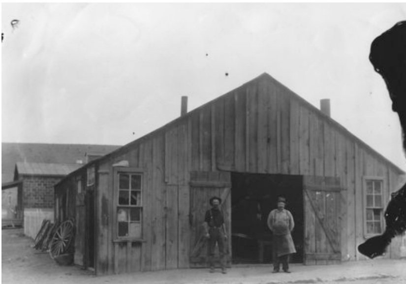
Photo 10: Blacksmith shop with Public Hall behind it
