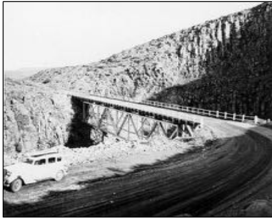
The Warren deck truss bridge over the Percha Creek box canyon, c. 1950. Note the "W" style trusses. Photo Black Range Museum.
