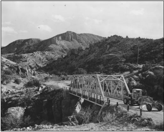
The second of the three truss bridges between Hillsboro and Kingston, c. 1950., with “N” style trusses. Photo Black Range Museum.
