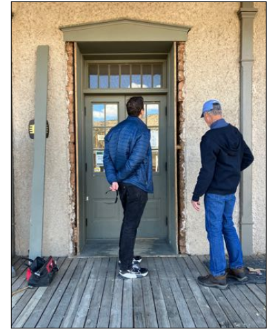
Site Manager Oliver Horn and Rand Berger examine the “notch” in Courthouse doorway made to accommodate the Mountain Pride in 1982.
