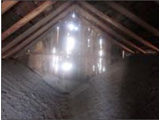
Fig. 11: Inside the attic over the BRM west section, 2017
