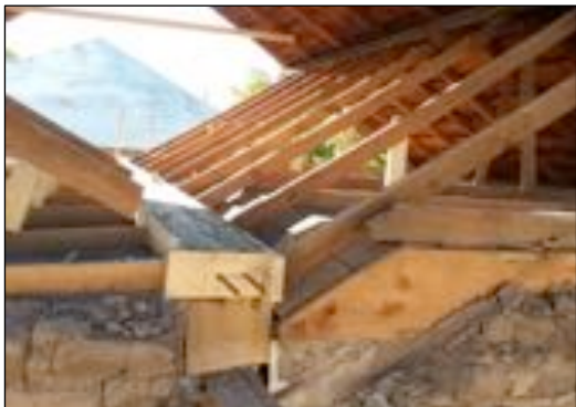
Fig. 22: New bond beam on top of wall dividing rooms
