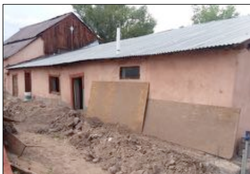
Figs. 15 and 16: (Left) Steve Dobrott clearing debris after removal of latillas and mud ceiling (Right) Mud from the ceiling piled outside the building
