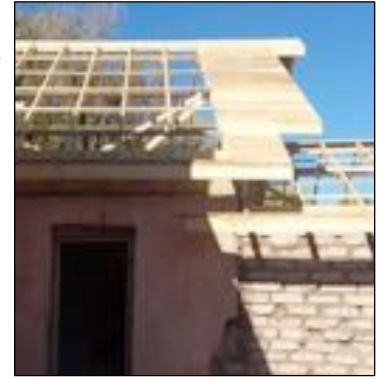
Fig. 23: Roof over the irregularly shaped rooms of the west section
