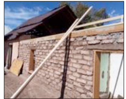
Fig. 20: Rebuilt adobe walls
