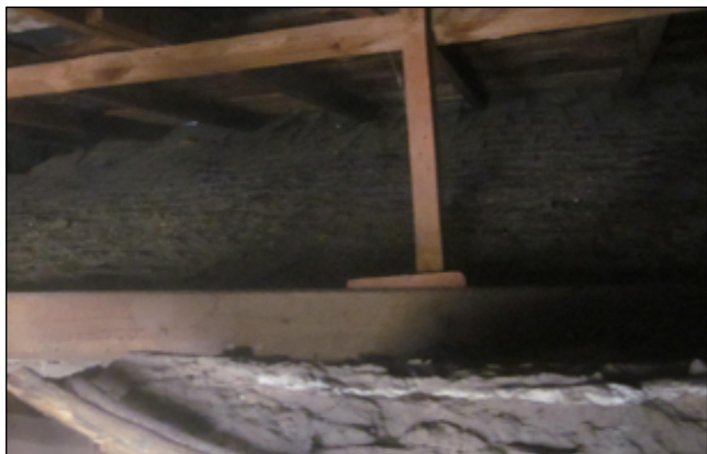
Fig. 14: Attic above Rooms 4 and 6 with latillas and mud forming original roof
