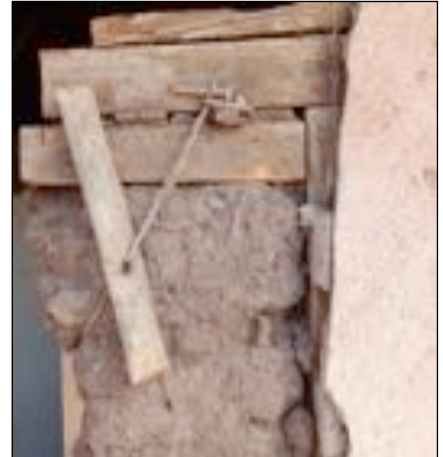
Fig. 18: The winding board tightening the joining of two walls
