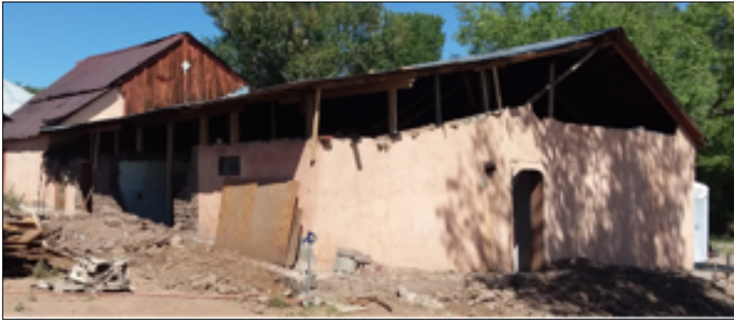
Fig. 19: Literally raising the roof on the east section
