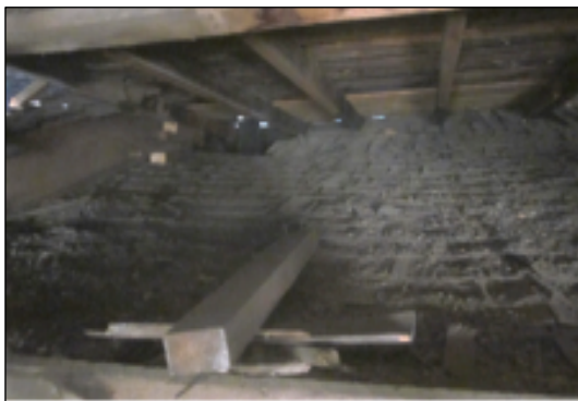
Fig. 13: In the attic of the east section looking north
