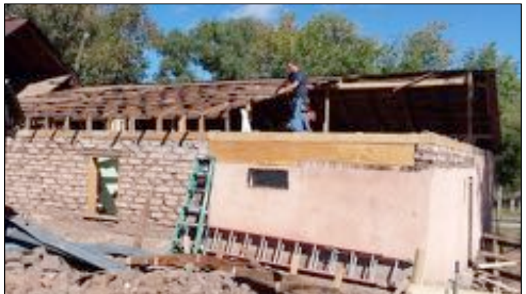
Fig. 21: Asa Cosper removing the old east section roof
