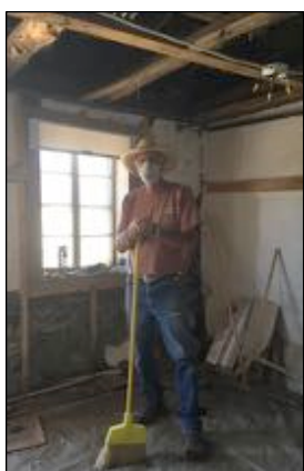
Figs. 15 and 16: (Left) Steve Dobrott clearing debris after removal of latillas and mud ceiling (Right) Mud from the ceiling piled outside the building
