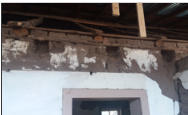
Fig. 17: North wall of Room 4, supporting the original roof
