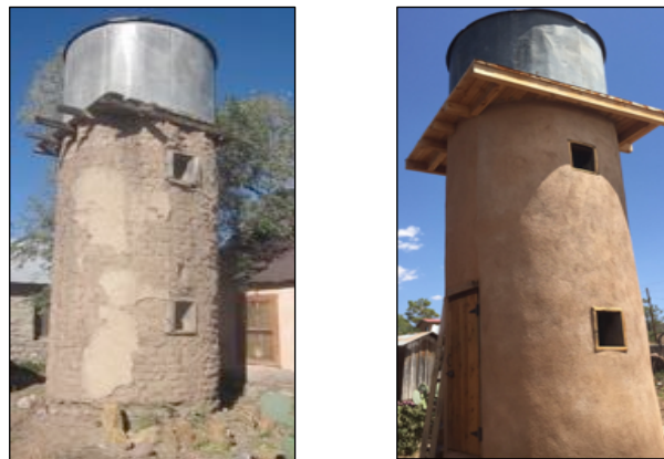
Figs. 4 and 5: Water tower before and after repairs
